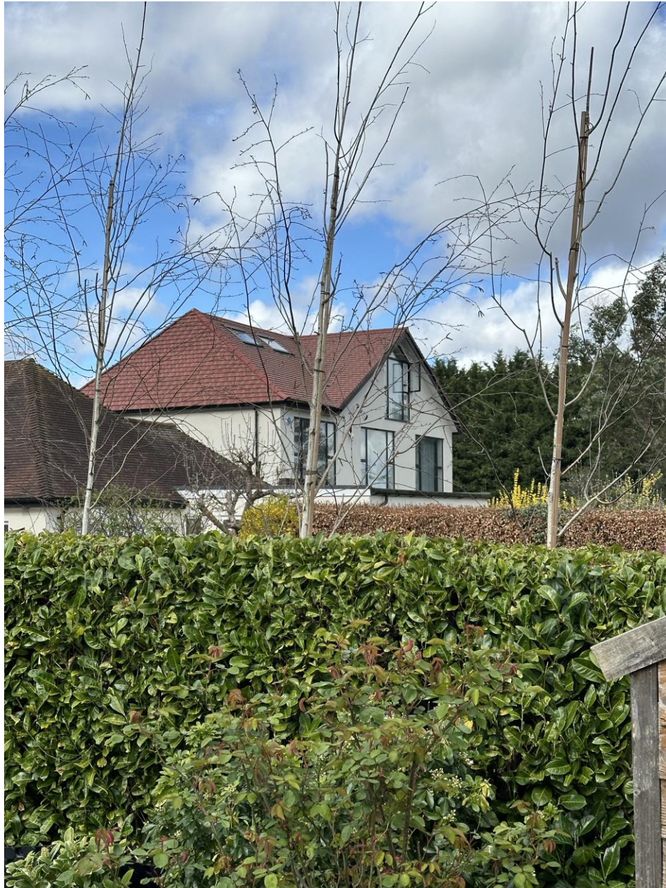
Figure 22 – Photo of Hillyfields (No.11 Hayes Mead Road)
